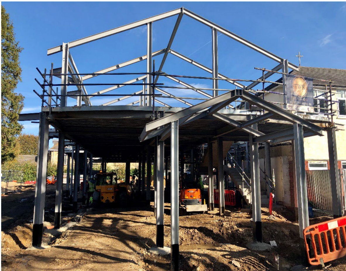
Picture: Integrated Rehabilitation Centre – Asset in the course of construction
